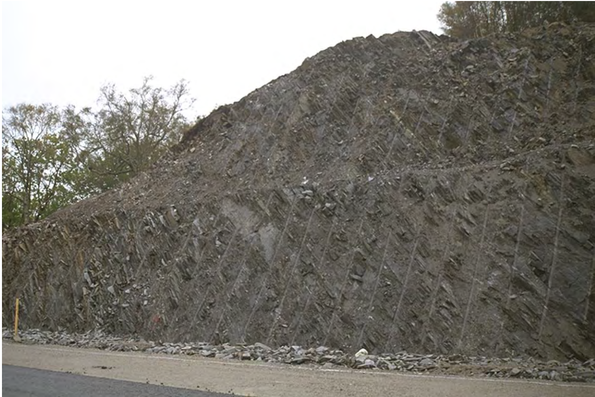
Figure 4. Pre-split rock cut slope on the A830 near Arisaig.
