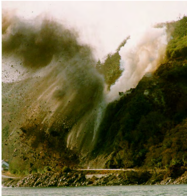
Figure 3. Rock blasting adjacent at the A83 Artilligan (image dated May 1997).
