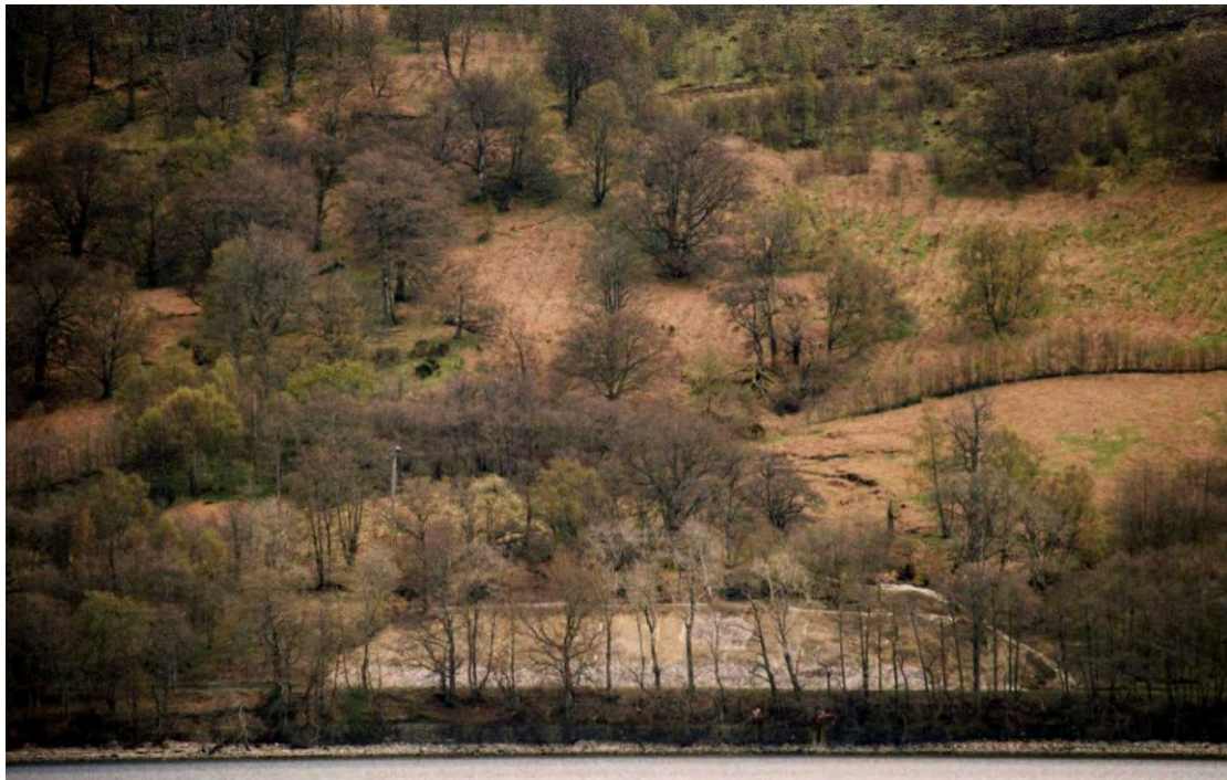
Figure 9. Translational landslide at A83 Loch Shira. The head of the landslide is located just below the middle of the image and above that point former plough lines left over after forest harvesting may be seen. (Image dated 1995).
